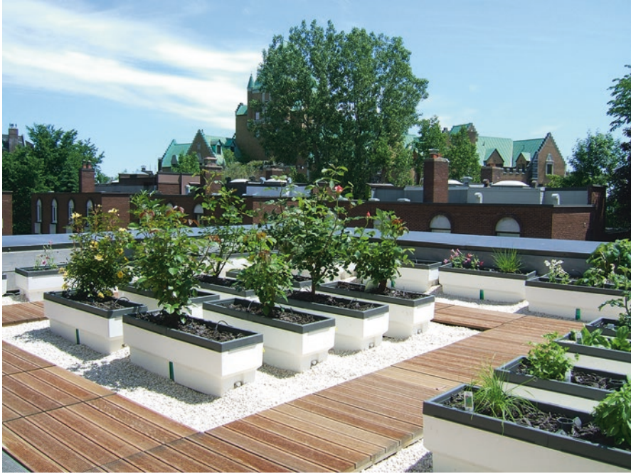
Fig. 3 Self watering planter with a water reservoir below the soil. (Photo: Courtesy of Bio Top)
