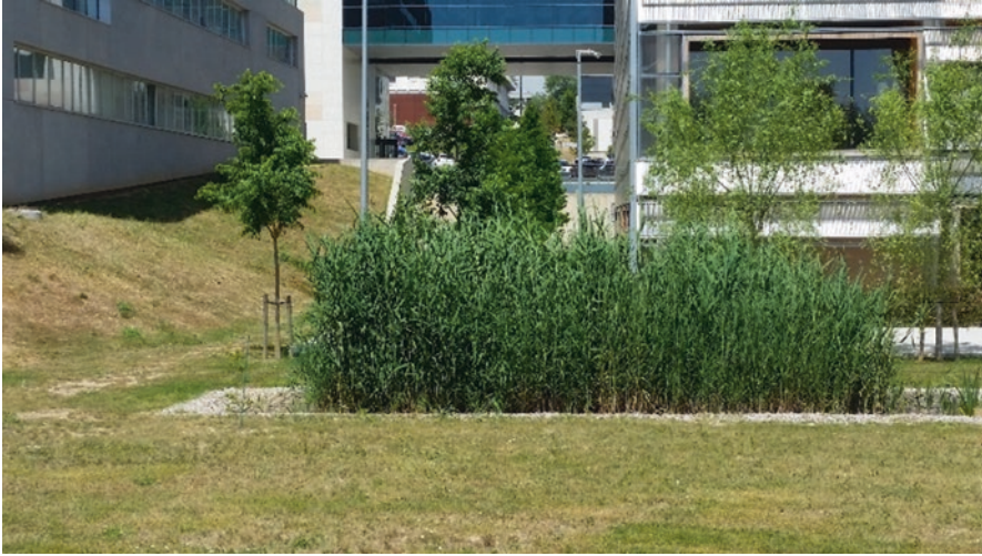
Fig. 8 Wetland for lixiviate treatment in ICTA Building, Barcelona, Spain (Photo: Sostenipra Research Group)
