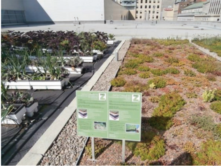
Fig. 34 The biotope-type planters ( left side ) and the green roof vegetation (Credit: Joe Nasr)
