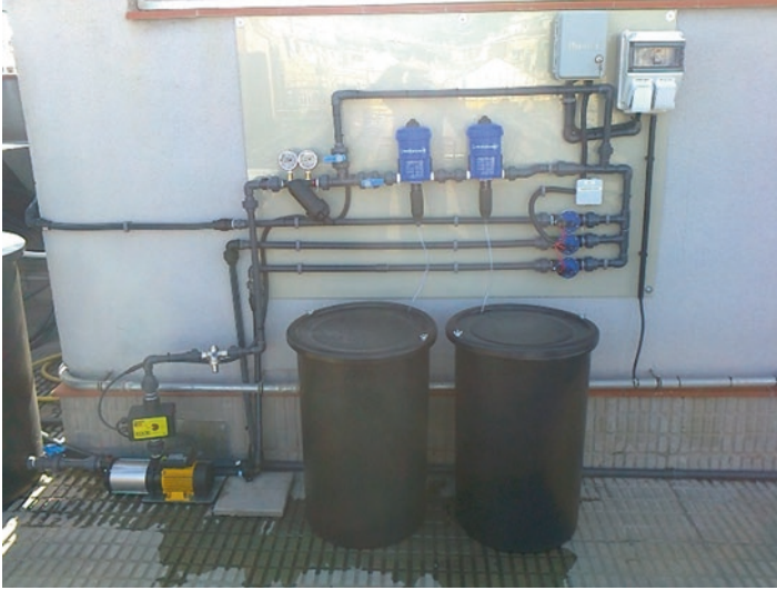
Fig. 6 Fertigation system with a domestic programmer, concentrated nutrient solution tanks and hydraulic injectors in an urban orchard in Spain (Photo: P. Muñoz)
