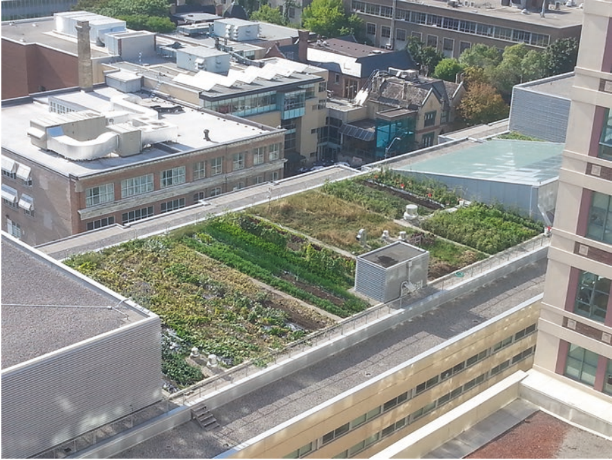
Fig. 1 Ryerson University in Toronto converted an extensive green roof into an urban rooftop farm. (Photo: A. Throness)
