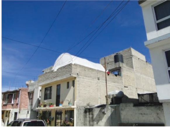
Fig. 46 The rooftop greenhouse established by one of the trainees, Daniel Hernández Campusano, Colonia San Miguel, Toluca (Credit: Gloria Samperio)
