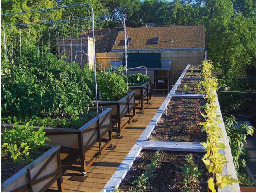
Fig. 2 Planters on the Uncommon Ground roof in Chicago are used as barriers for safety on the roof. (Photo: M. Cameron)
